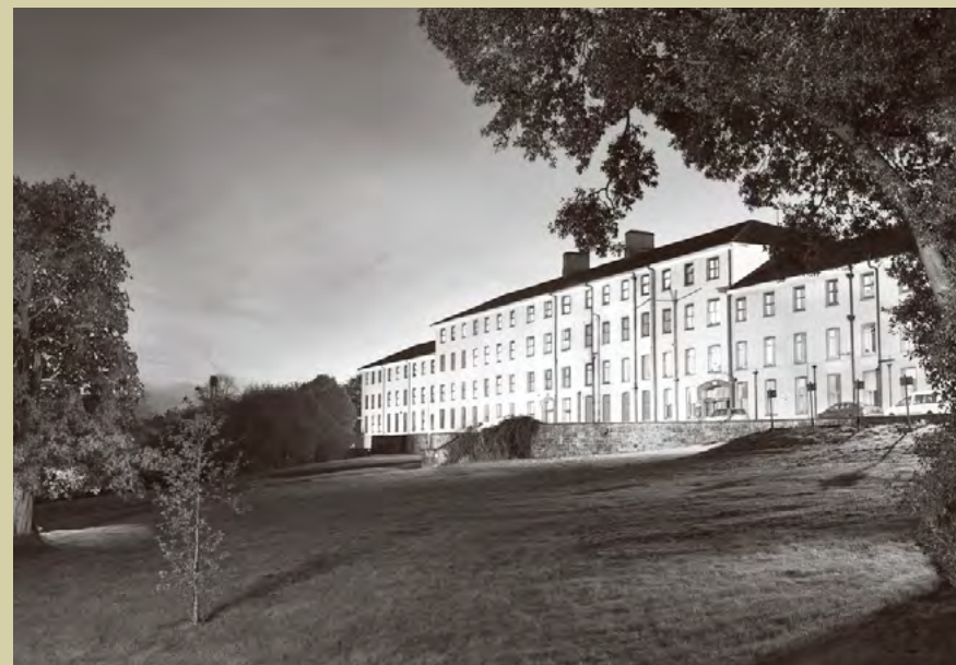
South Tipperary General Hospital
