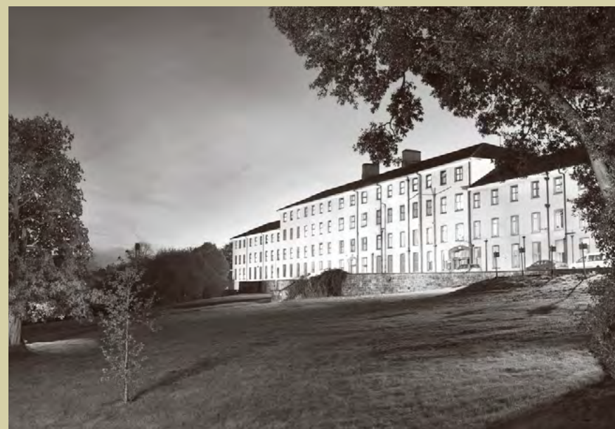
South Tipperary General Hospital
