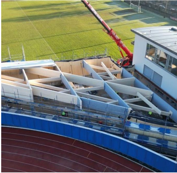
Fig. 10. Timber Frame installed in Mardyke
